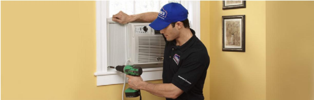
This system is technically called a “unitary” air conditioning system and consists of a self contained air conditioning unit that is placed in a window or through a hole in an exterior wall.
